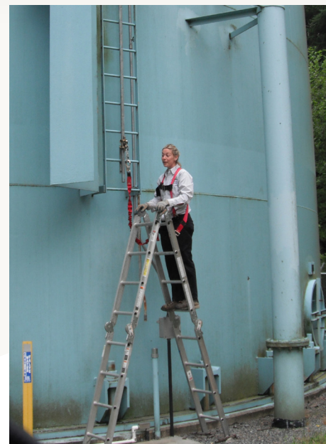
Amanda Worzella, an operator at Cross Valley Water District, gears up for an annual inspection of the standpipe.
