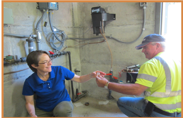
Sanitary surveys help us understand how water systems deliver water to customers. Here Nancy Feagin, surface water program engineering specialist, and Mike Williams, lead operator, test Sultan Water's combined filter effluent turbidity.
